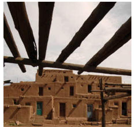
North Building of Taos Pueblo, Taos, New Mexico
